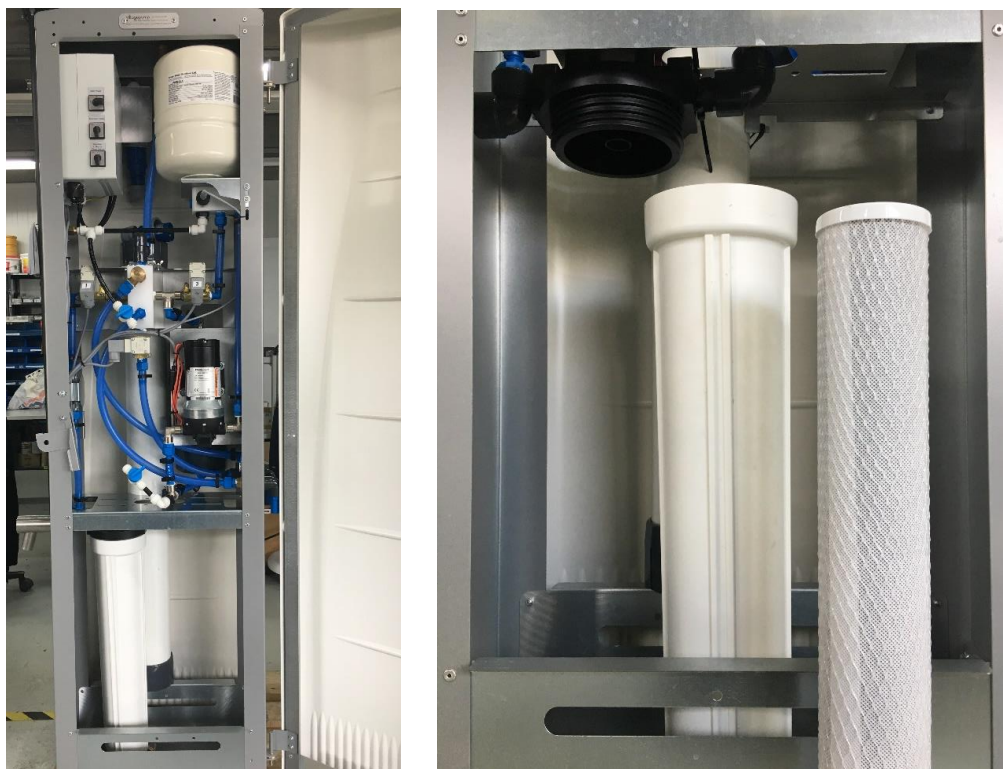
Installing AC filter cartridge: 2,5"x 20"
